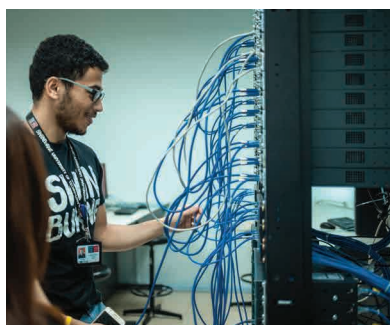
Our CISCO accredited training laboratories enable you to build large-scale broadband networks
